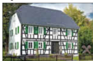
Raiffeisenhaus in Flammersfeld
